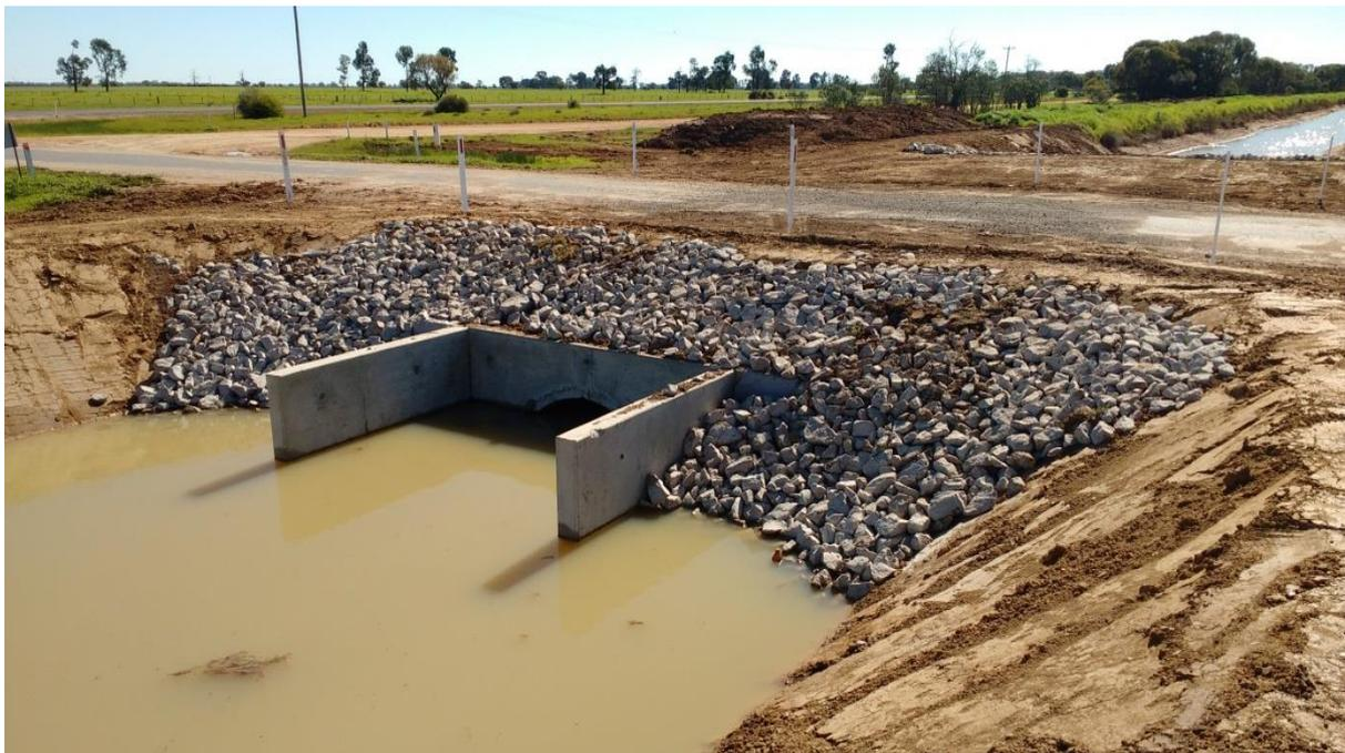
**Photo 2 - Upgraded regulator to overcome a previous channel constraint**
