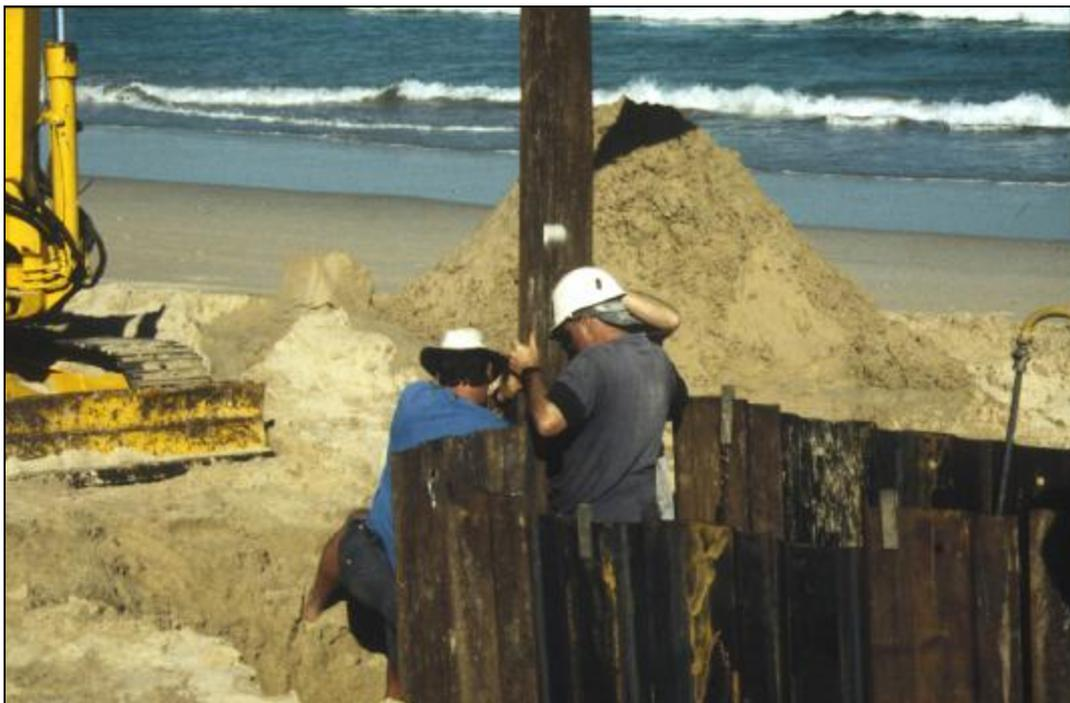
*Figure 10: Backhoe removed overburden of sterile sand and drove home the sheet piles.*
