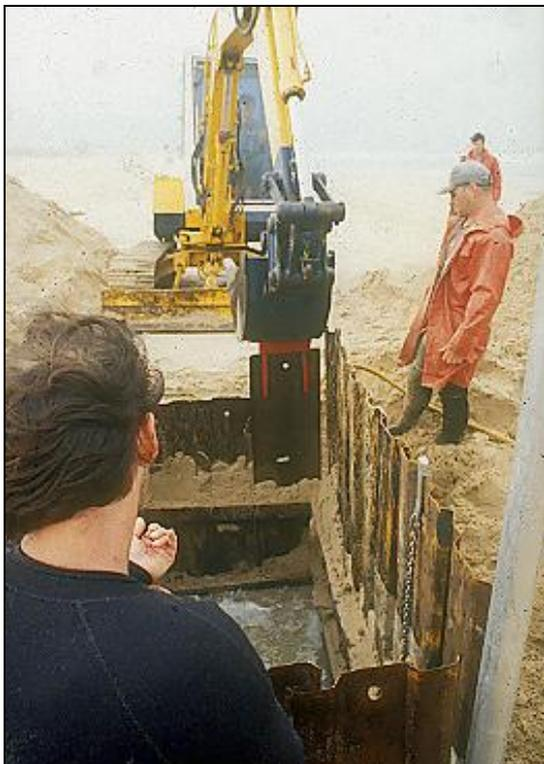
*Figure 11: Hydrated sand below the water table moved to refill the excavated caisson, leading to subsidence in the surrounding area.*
