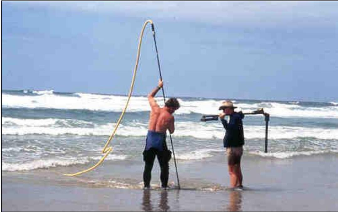
*Figure 9: A 4m compressed air probe was used to accurately place the corners of the caisson in relation to the iron object under the sand.*
