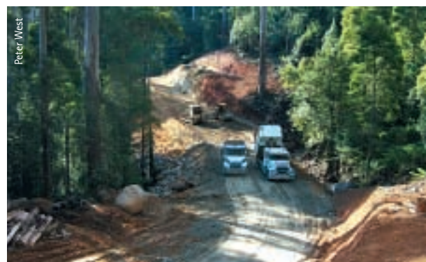
Construction of the South Face Road, Victoria
