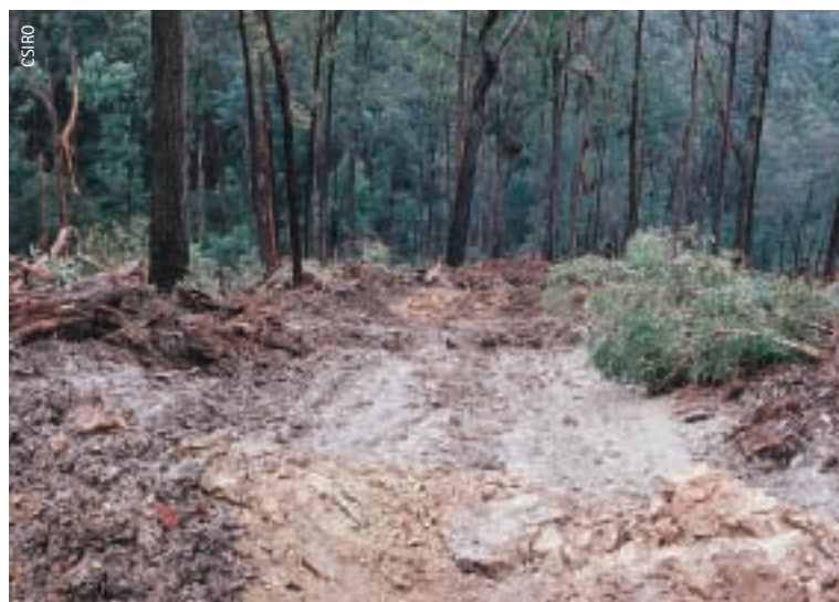
Snig track with erosion control barriers
