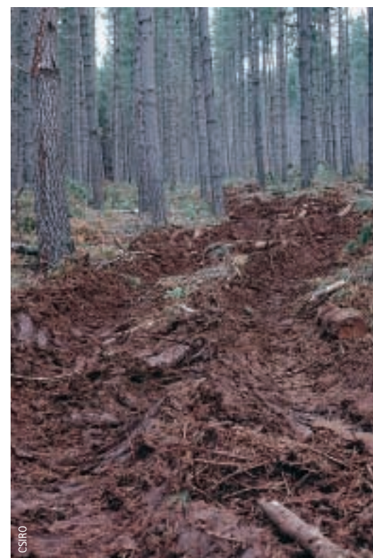
Cording of snig track to avoid rutting by machinery
