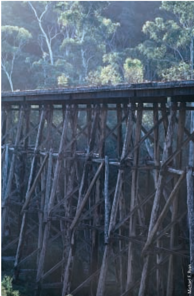
Timber trestle bridge
